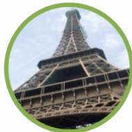
Eiffel Tower, France
